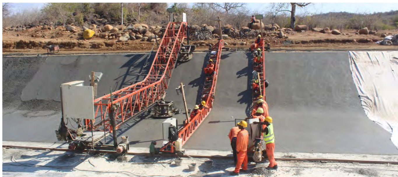
Civil Engineering students take part in the construction of Shire Valley Transformation Programme Canal (Irrigation Project) in Chikwawa District
